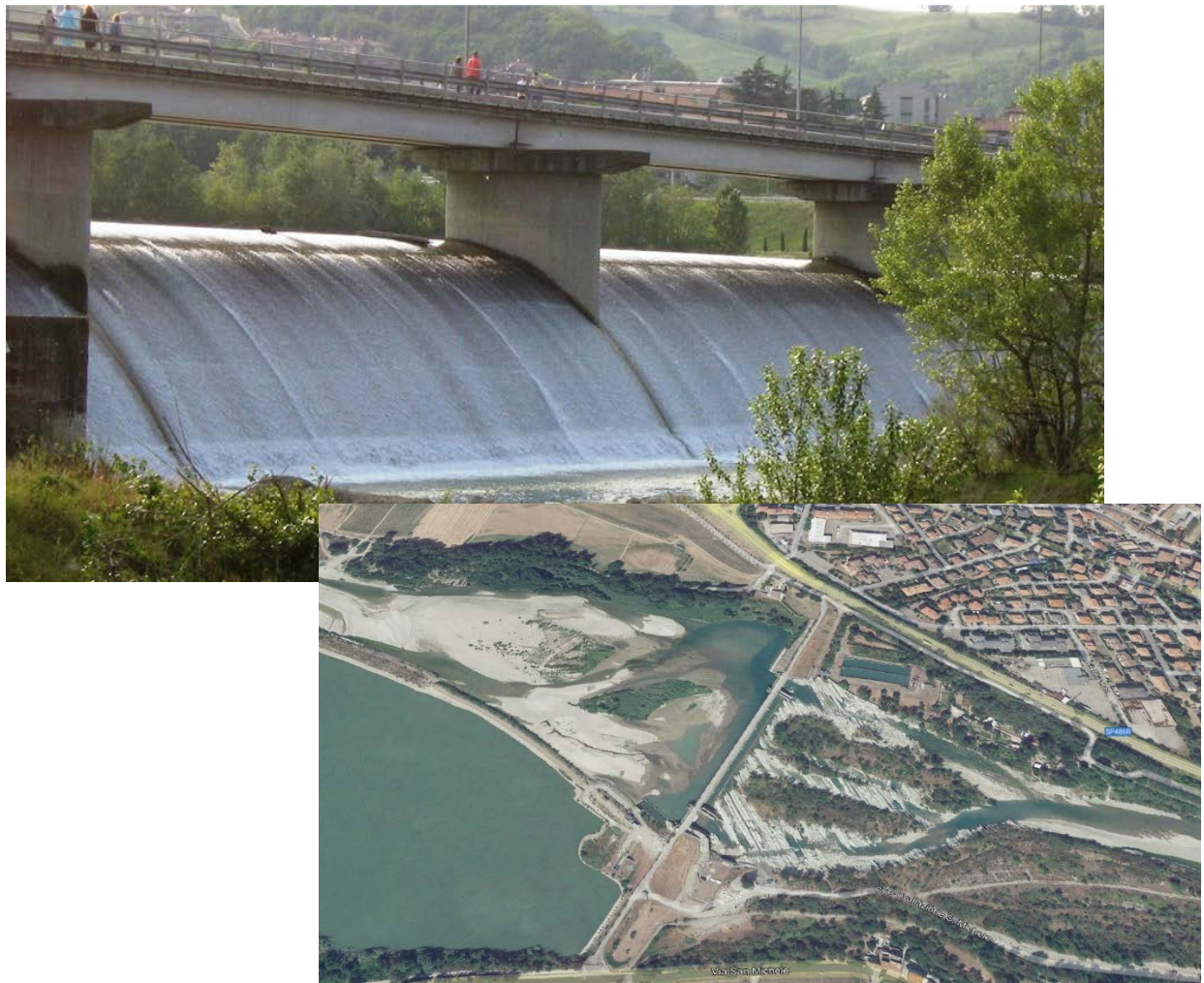
Figure 8. A view of the Weir at Castellarano along Secchia River
